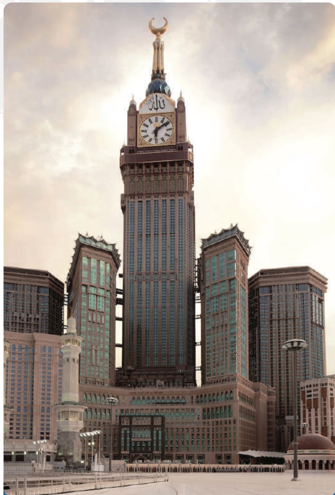
FAIRMONT CLOCK TOWER HOTEL MAKKAH
